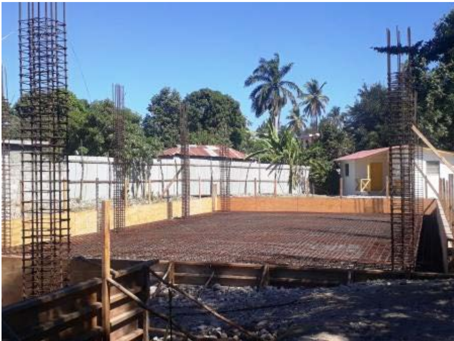
Finished reinforcement awaiting the pouring of concrete
