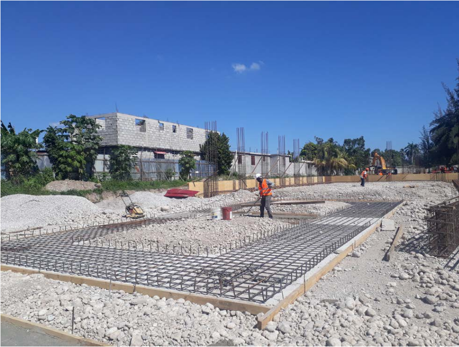
Finished reinforcement awaiting the pouring of concrete
