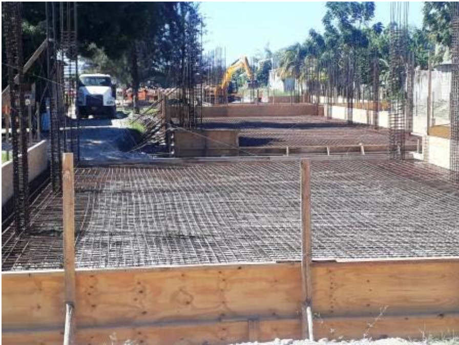
Finished reinforcement awaiting the pouring of concrete
