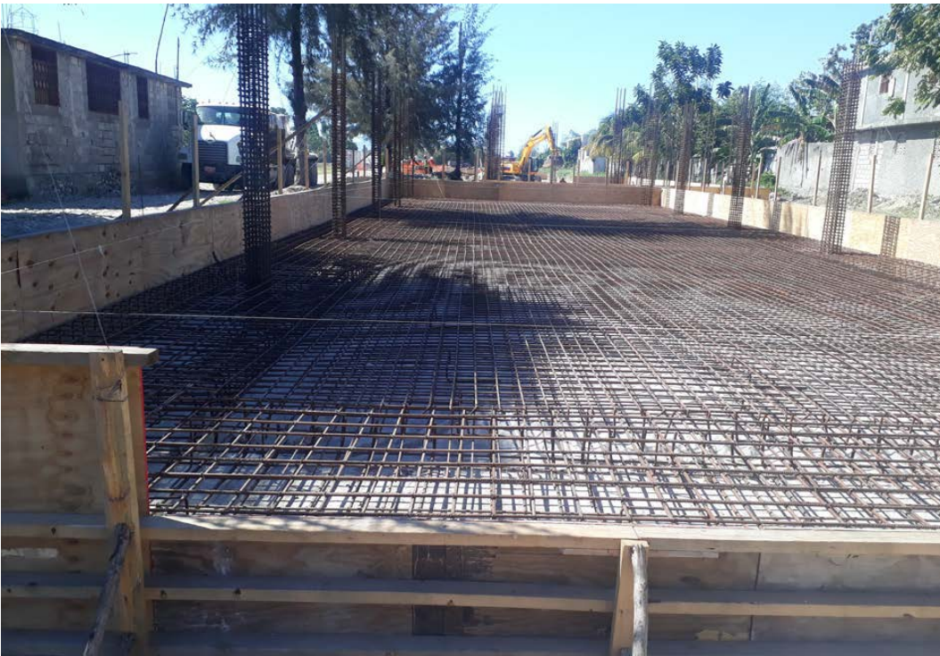
Finished reinforcement awaiting the pouring of concrete
