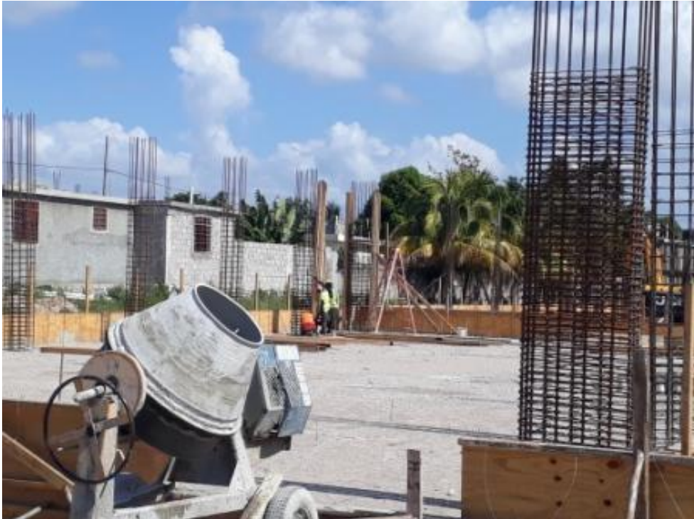
Les Cayes Works – Feb/2020
